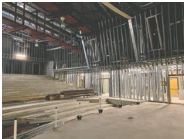
Stage left view of stage right construction work.
