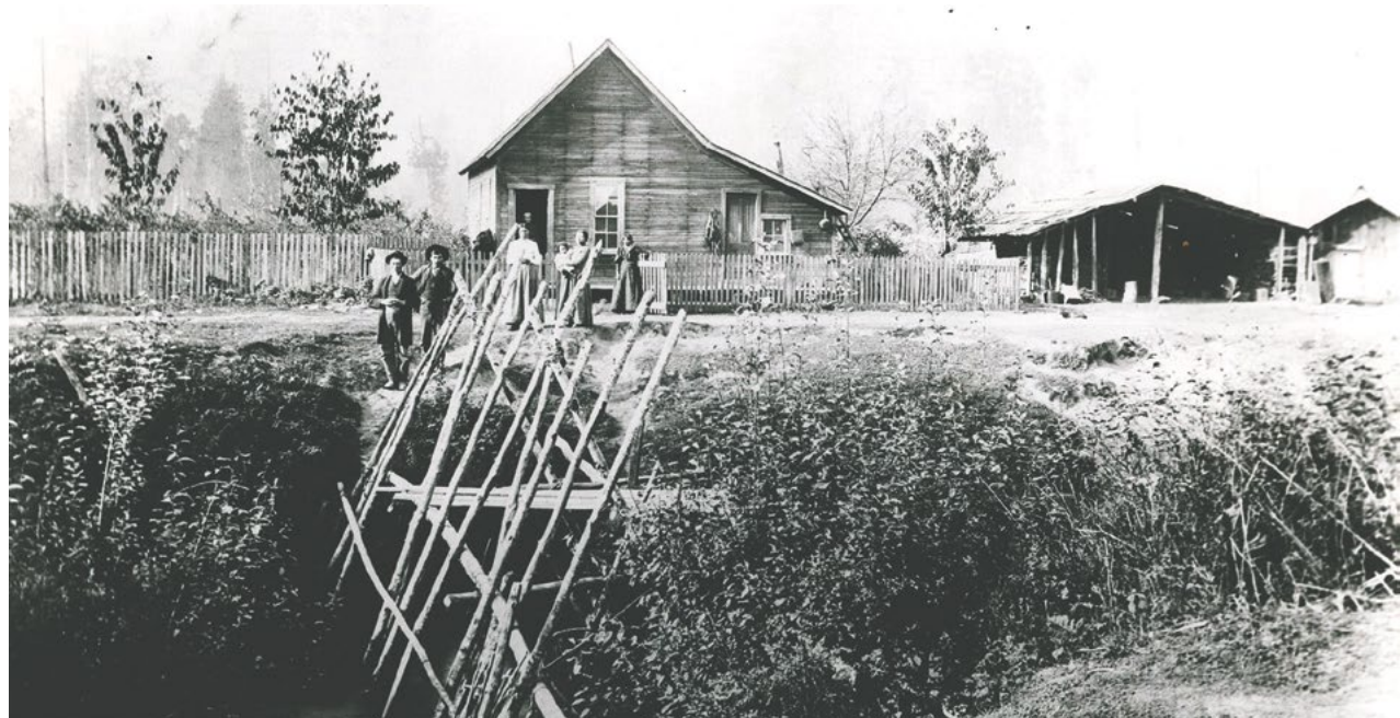
Photo provided by State Capital Museum, 1880's, unknown photographer. Small fishing weir located on Yelm Jim's allotment.
