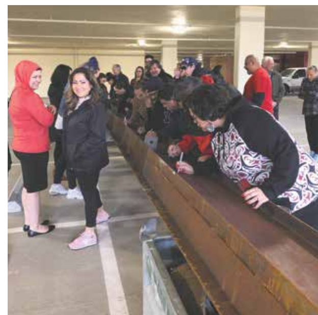
Puyallup Tribal Council member Anna Bean (front right) joins many others in signing the final beam for the new garage and hotel on Feb. 7.
