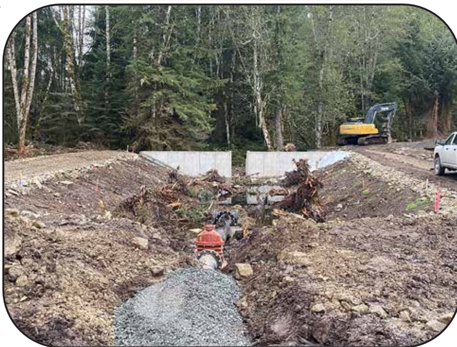
The re-engineered Rushingwater pond under construction during the summer of 2023.
