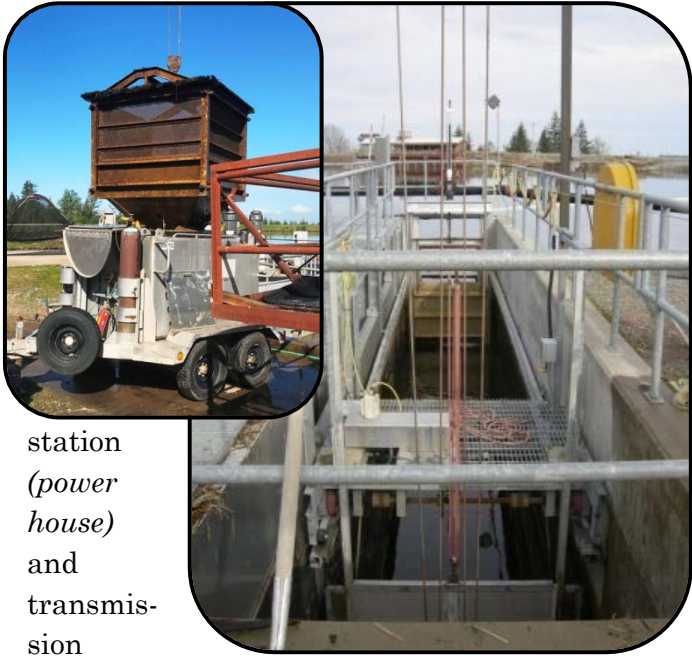
Electron Hydro fish collection facility (trap), and water-to-water fish transfer into hauling trailer.
