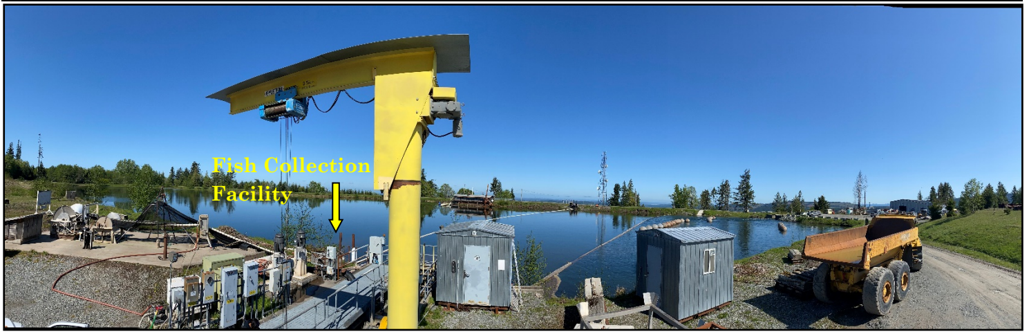
Electron forebay, and location of the fish collection facility.
